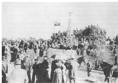
Laying of the University Hall's Cornerstone in 1890
