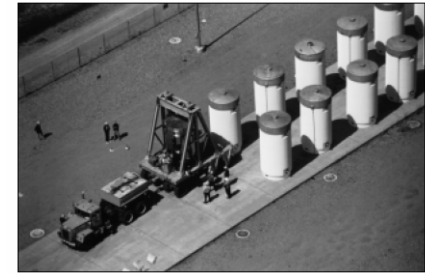
Concrete storage casks at a U.S. nuclear power plant (photo taken from Interim Storage of Spent Nuclear Fuel Report, June 2001)
