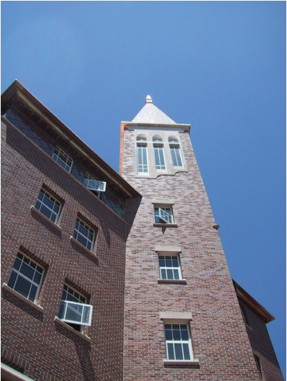
Nelson Residence Hall Tower
