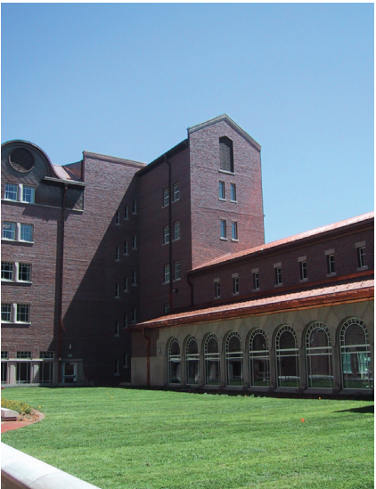
Nelson Residence Hall Courtyard
