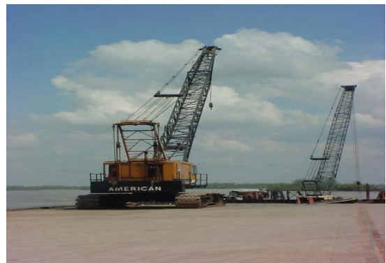
Figure 9. 125-ton capacity crane
