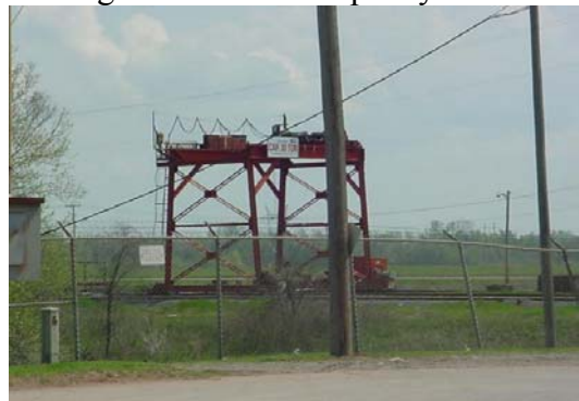
Figure 11. Rail-mounted gantry crane
