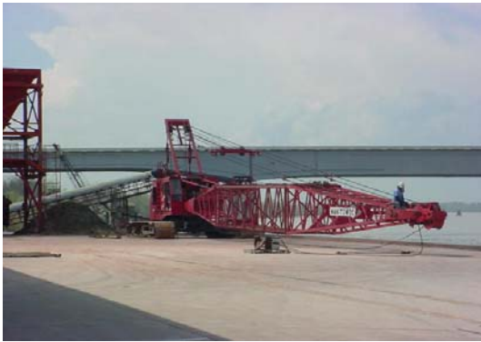
Figure 8. 175-ton capacity crane
