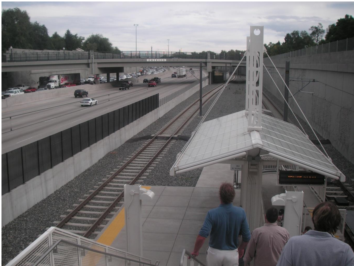
Plate 4.2 Louisiana-Pearl station on RTD's South East Corridor Light Rail line (photo © Andy Jonas, September 2007).
